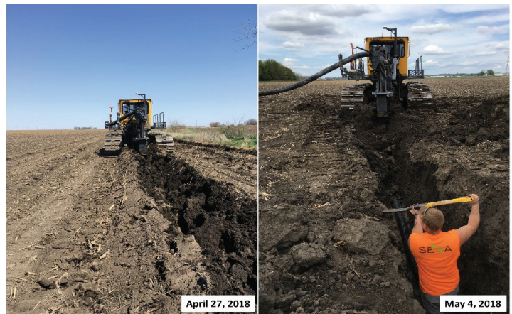
Tile being installed in the monitoring fields.
