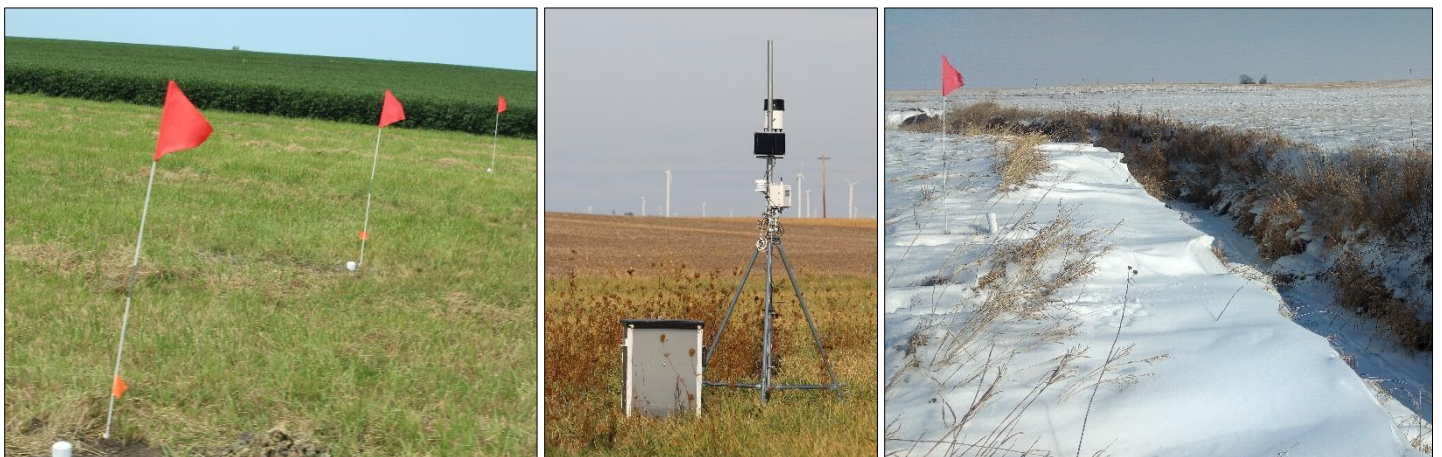
Figure 3. Sixteen wells and a weather station have been installed at the Knox County saturated buffer.
