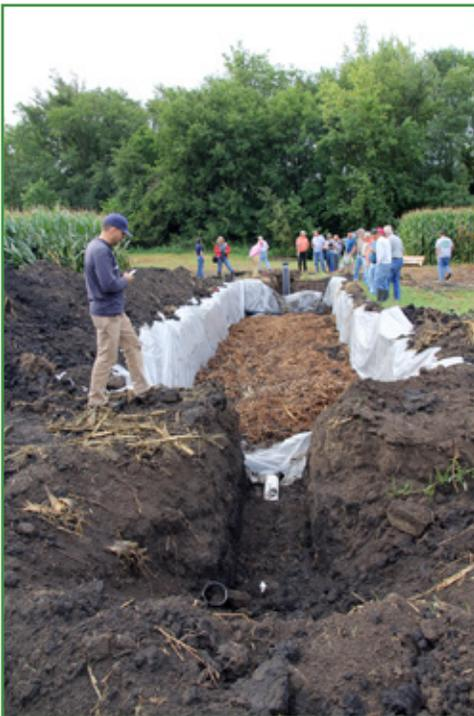
*This long view shows the bioreactor hole, lined with plastic and filled with wood chips. The bioreactor will then be covered in soil.*
